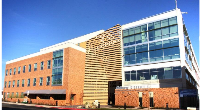
District 3 Headquarters, Marysville, CA
