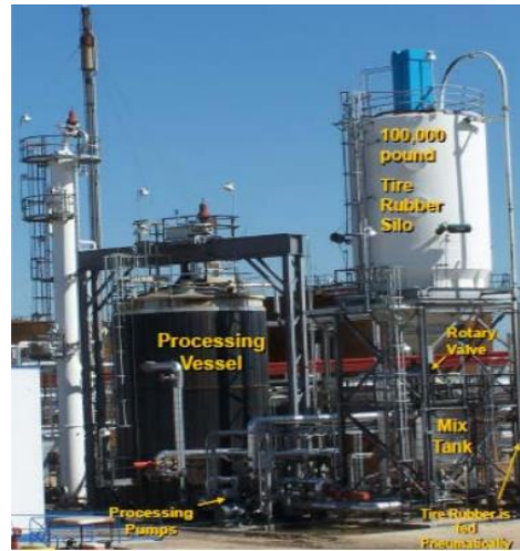
Terminal Blending Process for Rubberized Asphalt
